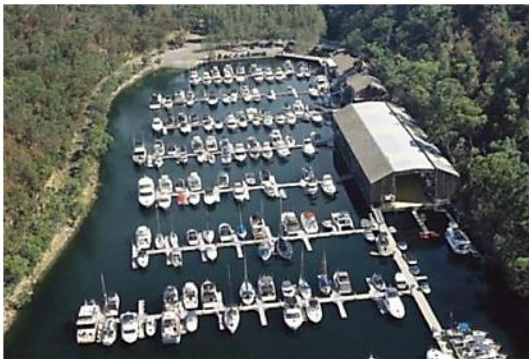
Figure 38. A typical marina in New South Wales
