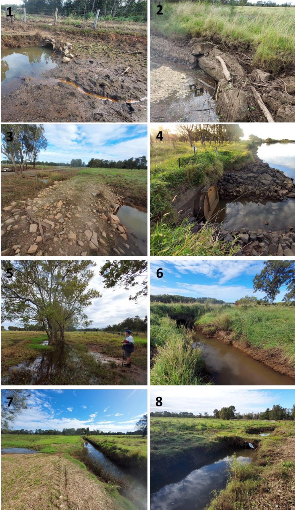
Figure 1.6 Georeferenced photographs showing the drainage channel network, end of drain culverts, tidal floodgates, and relict mangroves inside the regional levee (photo #5). See Figure 1.5 for photograph locations.
